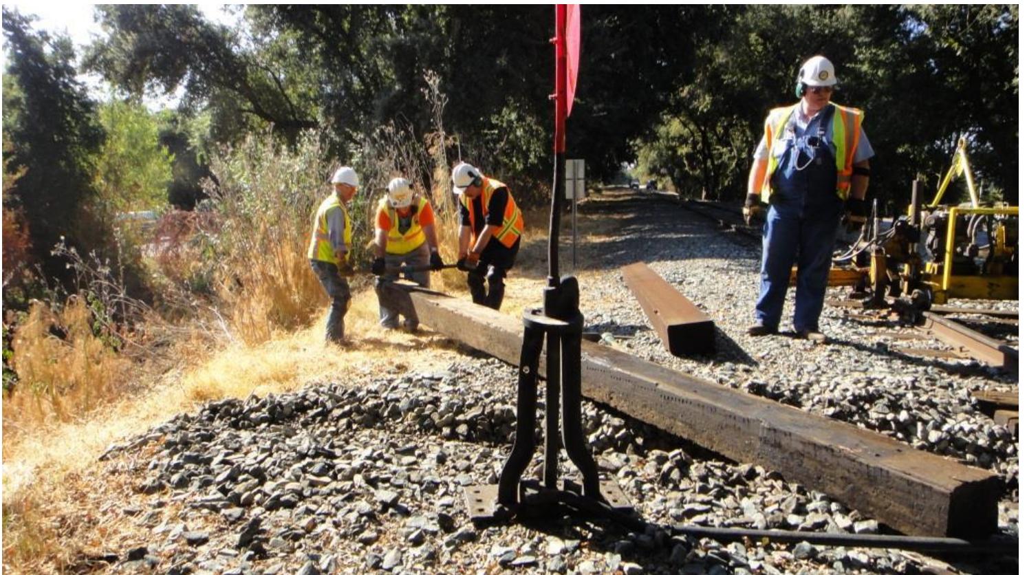
Now that the old head-block is removed, Mike T., Mike F., and Fred get it out of the way
