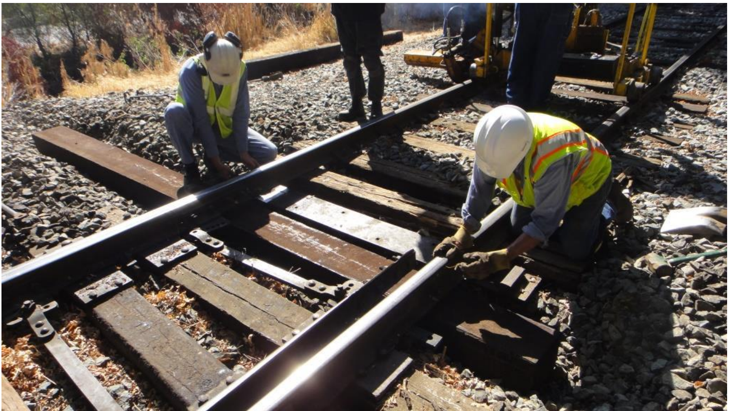
With the new head-block situated, Alan and Mike T., slide the gauge plate into place
