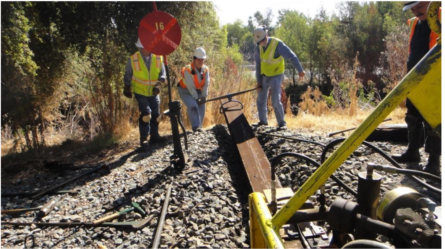
Heather and Alan guide the new head-block into place
