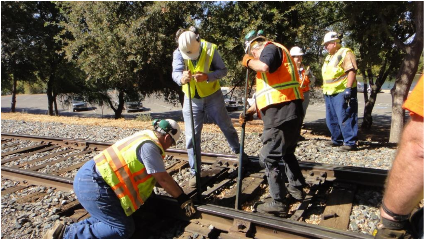
Let's get this right: Chris, Alan, and Fred move the east point to line the transit clip with the bolt-hole
