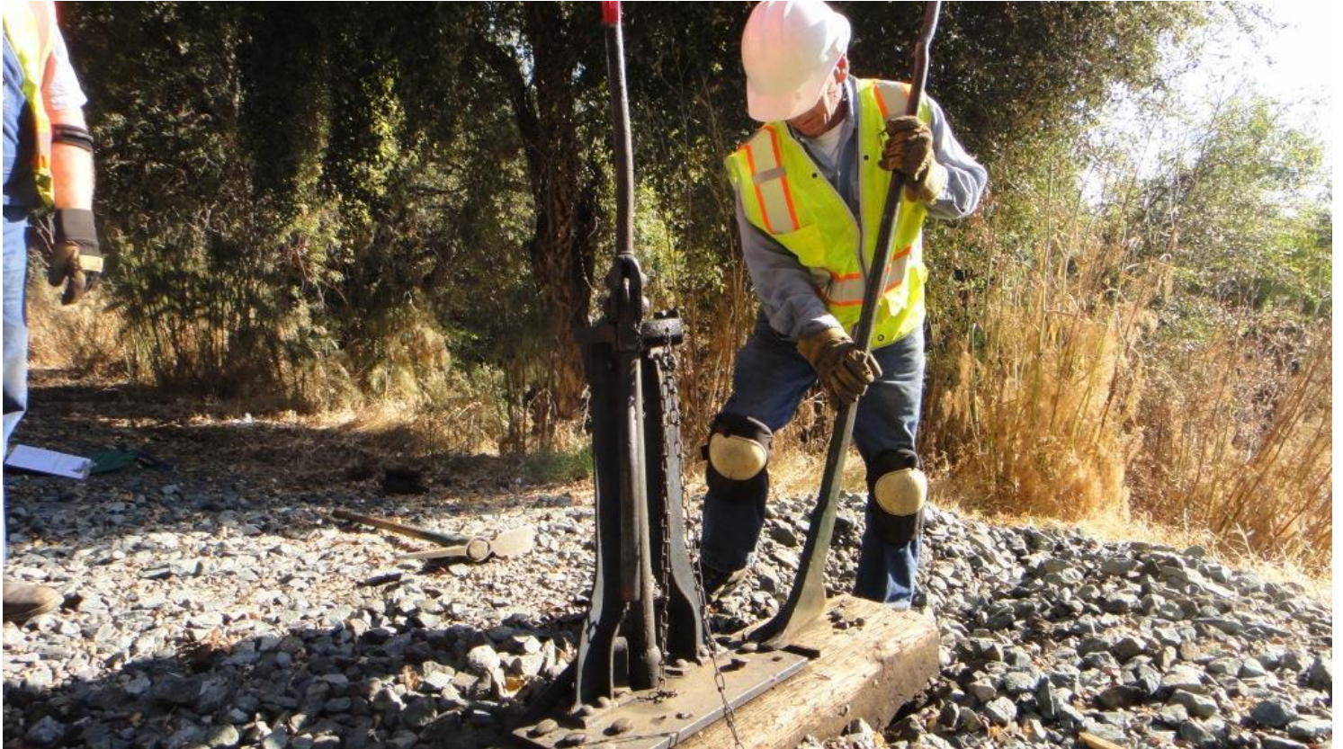
Mike T. removes the spikes from the switch-stand
