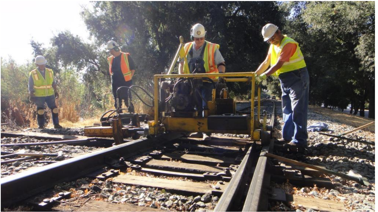
The section-gang machine makes quick work of removing the old head-block
