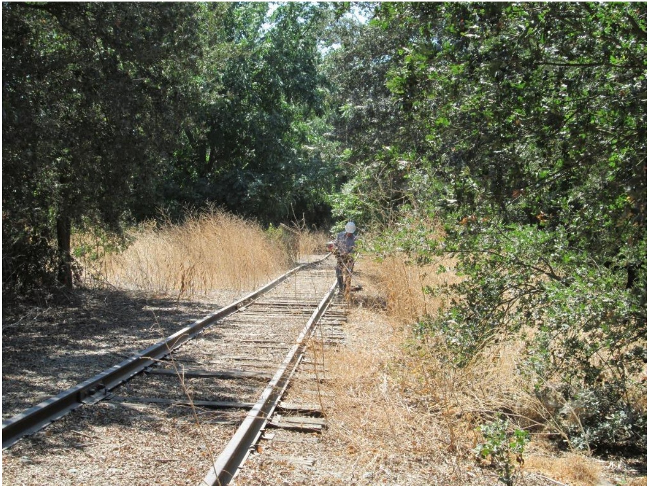
Mike T. clearing the right of way at Hood
