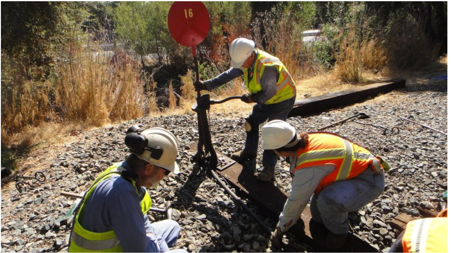
Alan, Heather, and Mike T., adjust the position of the switch-stand
