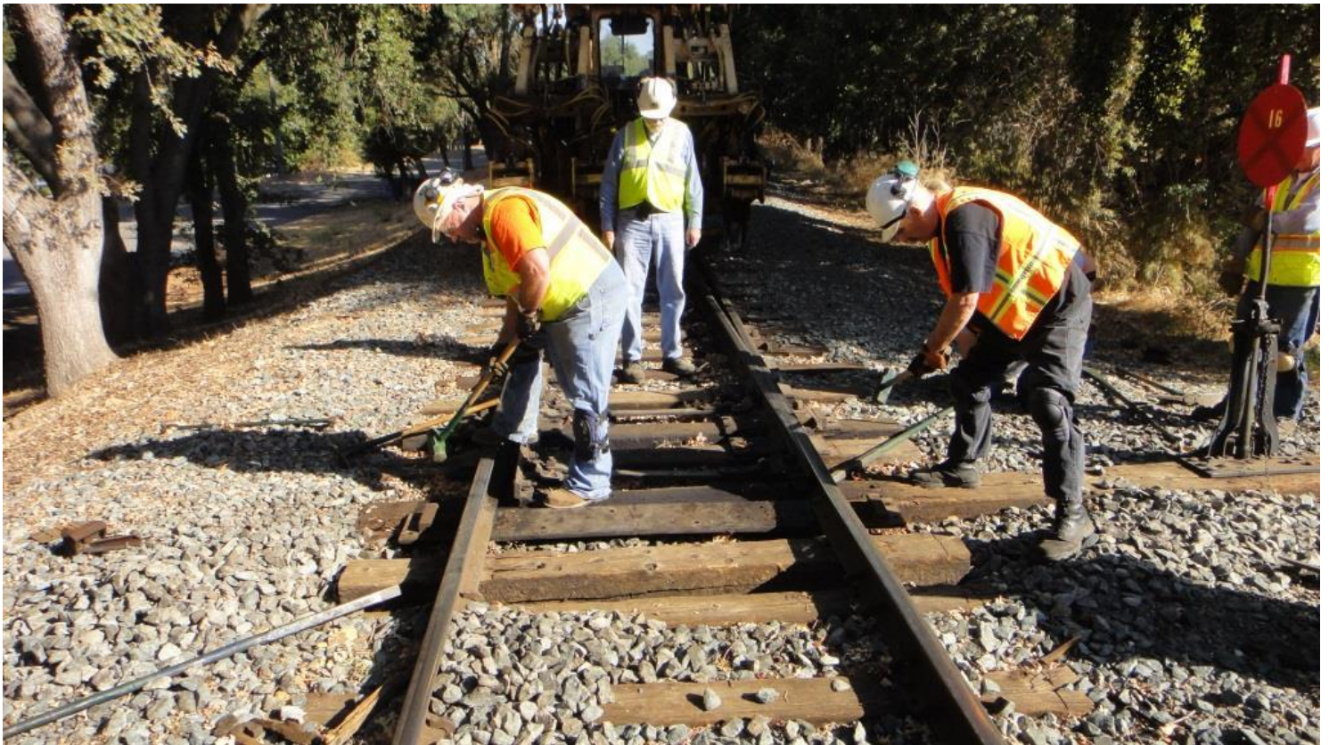
Mike F., and Fred shove the gauge plate off of the head-block and into the crib the adjacent tie
